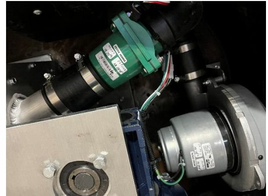
✓ New Blower & Plumbing
